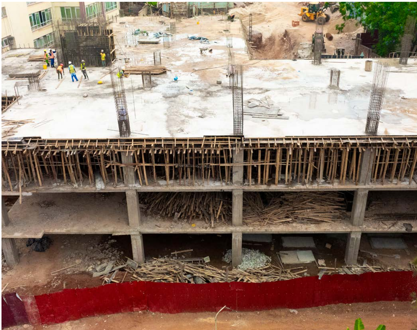
An aerial view of the new tuition block under construction.
